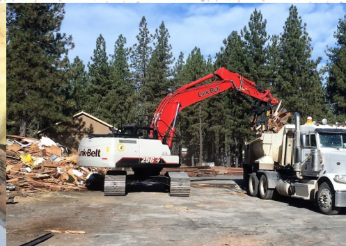
Building Demolition & Removal
