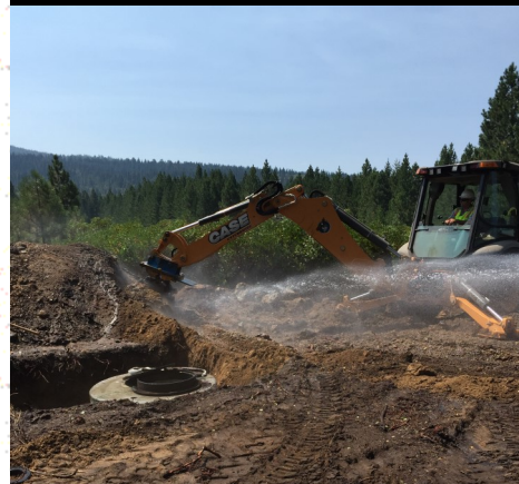
NPS—Manzanita Lake Sewer Replacement
